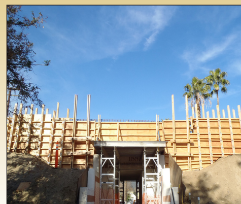
Formwork at the 5th Avenue pedestrian tunnel.
