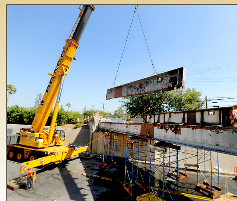
Removal of the old Colorado Bridge structure.
