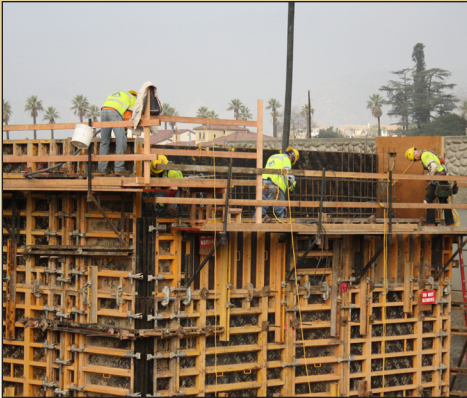
Abutment formwork at Citrus Avenue Bridge.
