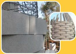
November 2012 was the last full month of construction work on the bridge. completed installation of the bridge "basket" features and retaining walls leading up to the bridge's two abutments. Additionally, crews began to pour concrete for the bridge barrier rail, the wall that rises above the bridge deck. Crews also removed various construction materials, such as the steel and wood used for the falsework, from the I-210 Freeway's center
