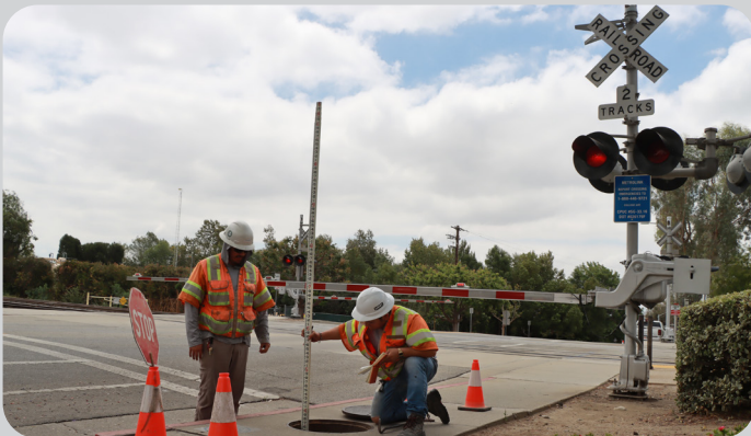
Surveying crew collecting data at College Ave. crossing in Claremont to inform project design effort by Parsons.
