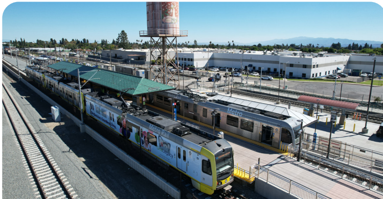
Four new Metro A Line stations from Glendora to Pomona are now open for passenger service. Pictured: Pomona North Station.
