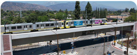
New light rail bridge over Bonita Ave./Cataract Ave. intersection in San Dimas.
