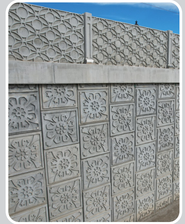
Sound Walls (top) and Retaining Walls (bottom)
