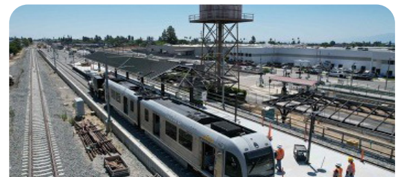
Crews pulling the unpowered light rail vehicle into the future Pomona station to conduct clearance testing.
