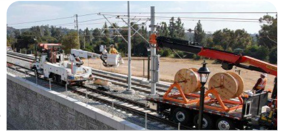
Crews completing final miles of overhead wires for the power system.
