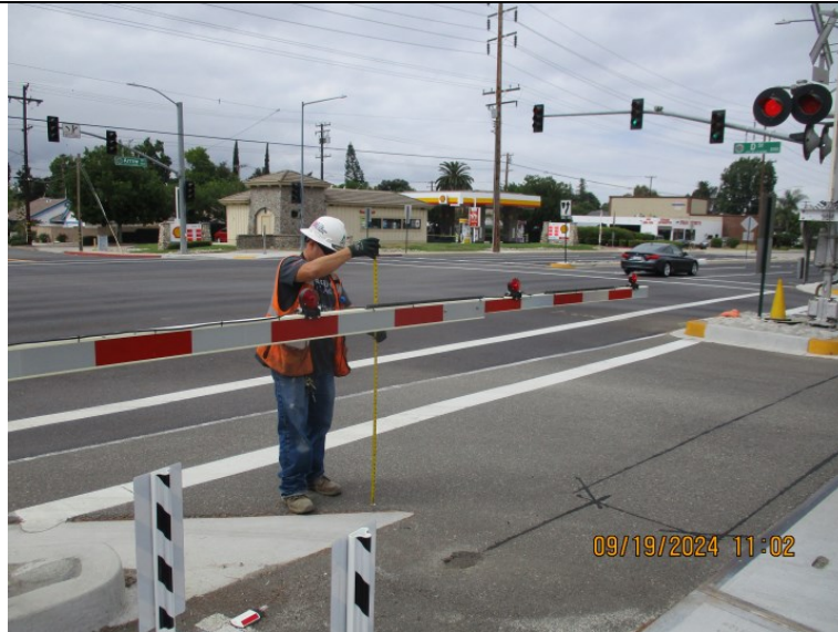
D Street - Monthly grade crossing testing
