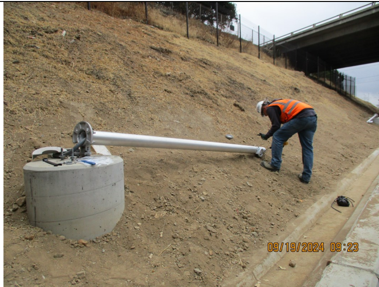
Route 66 to San Dimas Wash - CCTV utility poles
