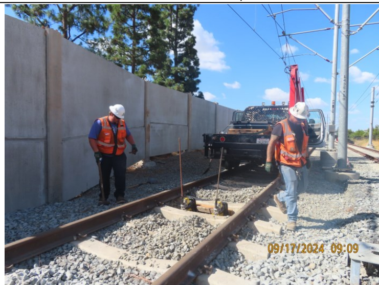
Glendora Station - CIC conduit adjustments
