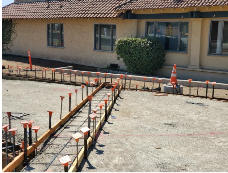
Glendora Station Plaza - Concrete ribbon curbs
