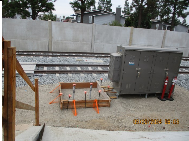
BOP - Disconnect switch pad formwork
