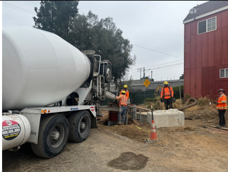
San Dimas Station Parking - Light foundations
