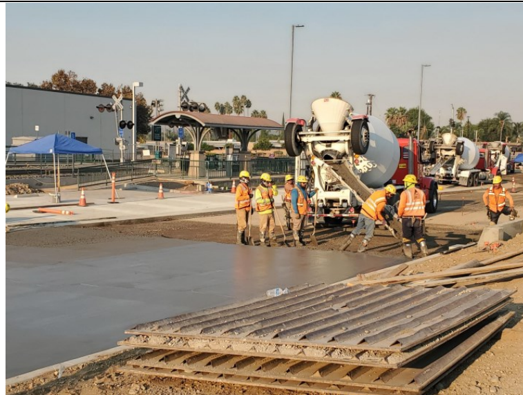
Pomona Station Parking - Concrete paving
