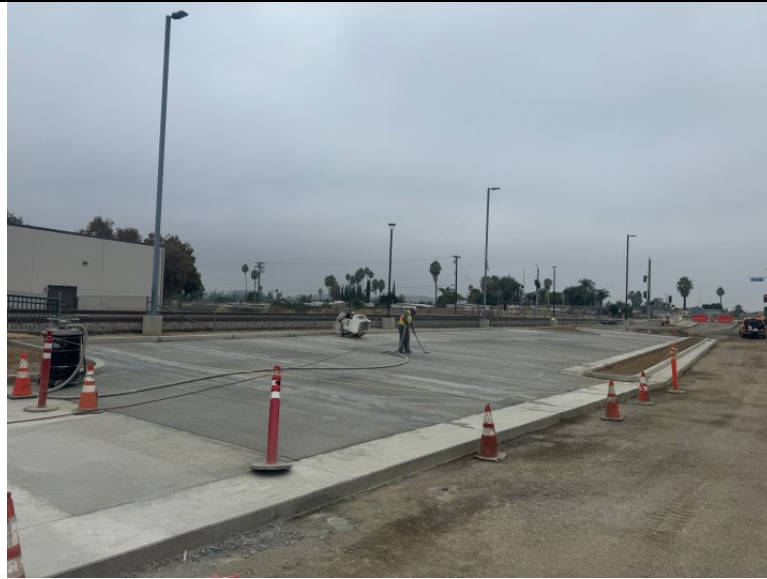
Pomona Station North Parking - Concrete sawcut
