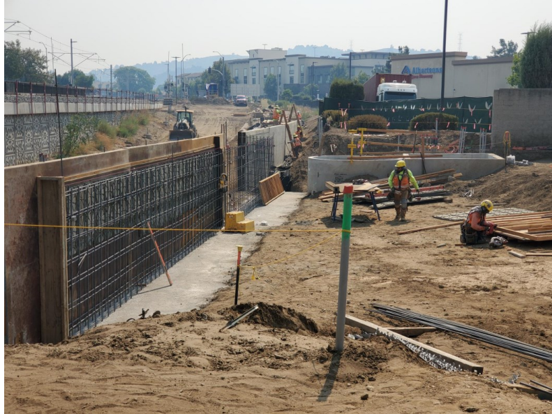
Glendora Station Parking - Retaining wall
