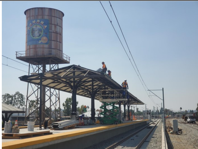
Pomona Station - Boarding canopy roof
