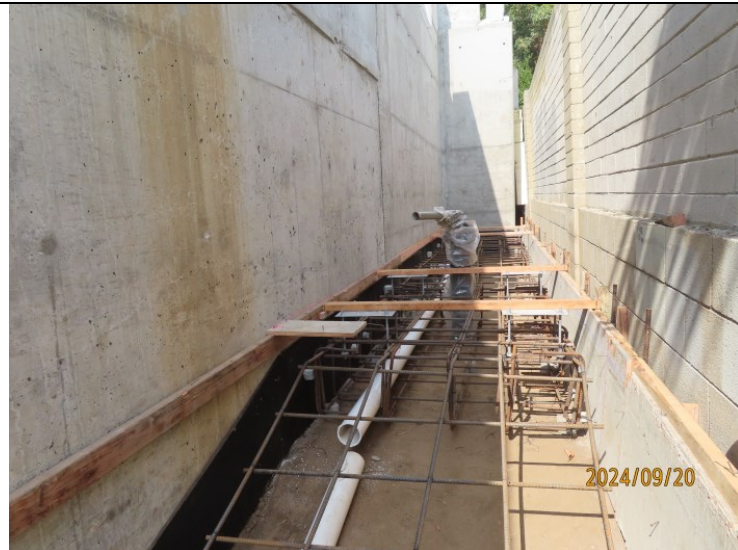
Route 66 - Emergency access stairs foundation
