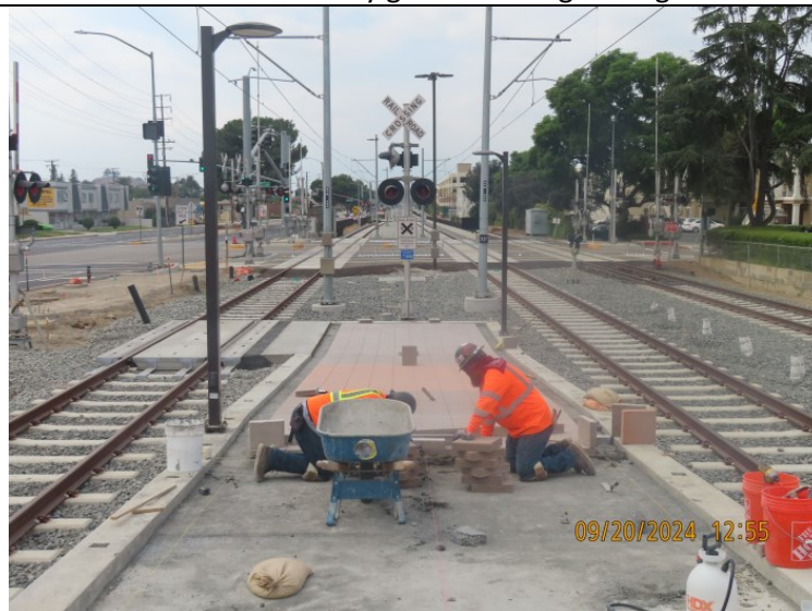
La Verne Station - West ramp pavers
