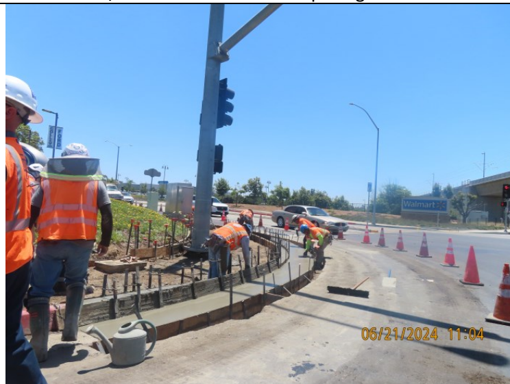
Lone Hill/Auto Centre - Curb and gutter replacement
