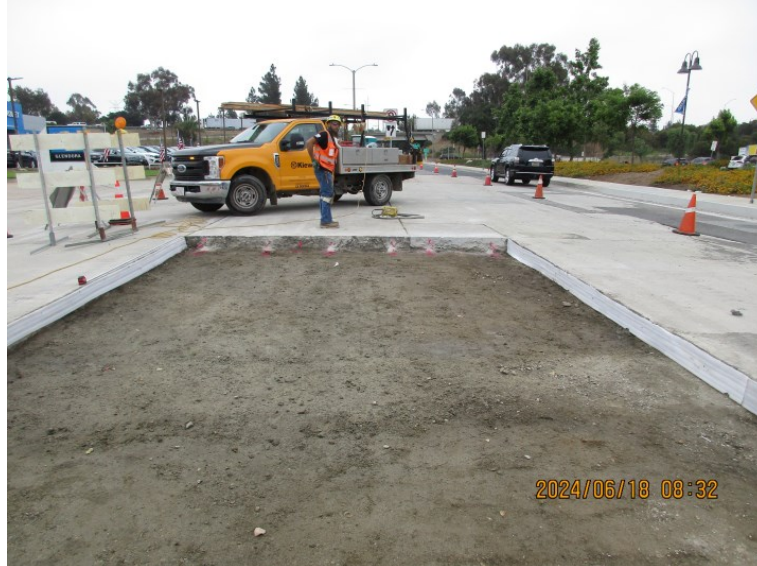
Lone Hill/Auto Centre - Concrete paving reconstruction
