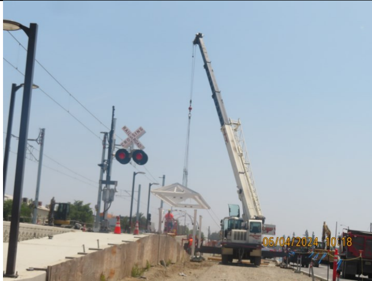
Pomona Station - East ticketing canopy
