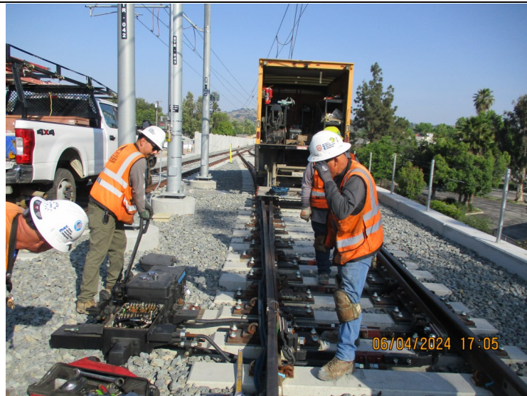
Carroll interlocking - Switch adjustment
