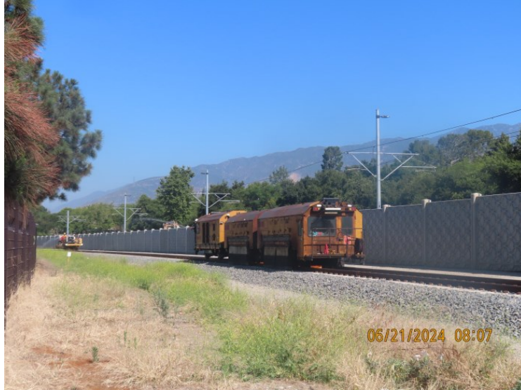
Barranca to Foothill - FRT rail grinding
