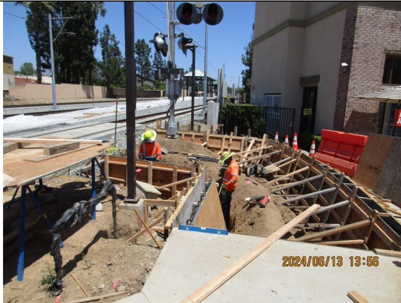
San Dimas Station - Entrance retaining curb
