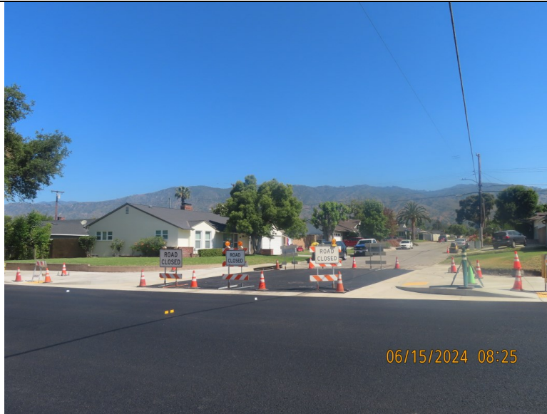
Elwood/Foothill - Roadway paving
