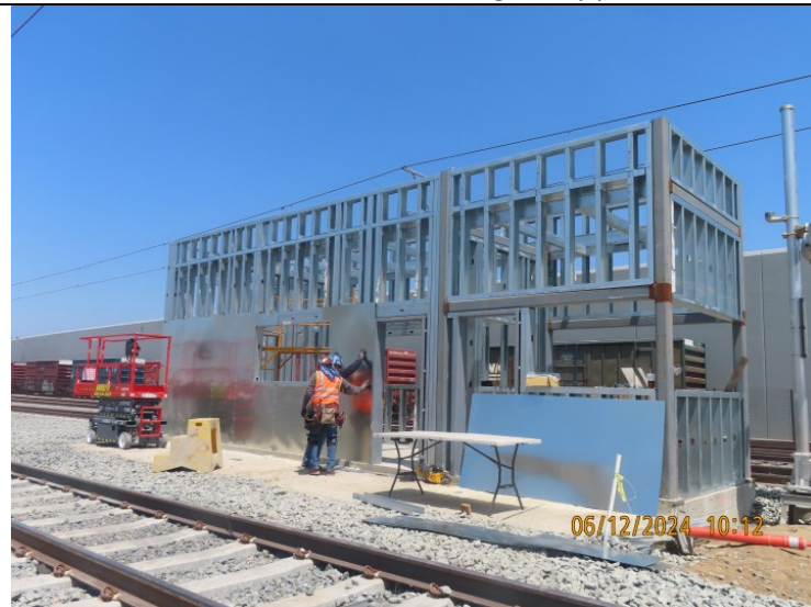
Pomona Station - Layover building
