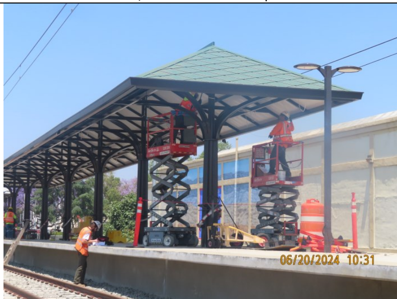
La Verne Station - System cable installation
