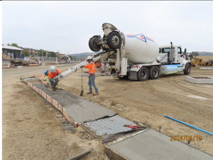
Glendora Station parking - cross gutter replacement
