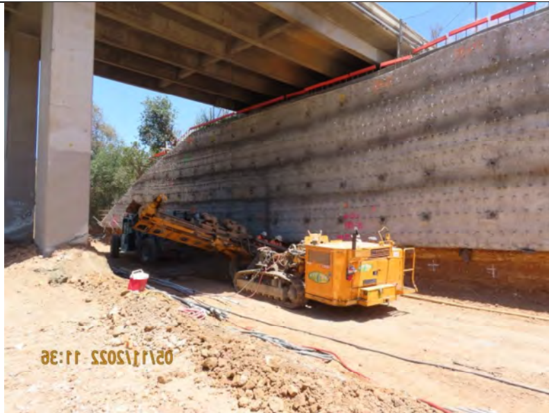
210 FWY—Ground anchor wall
