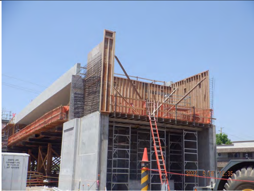
Bonita Cataract—LRT Structure wingwall and backwall
