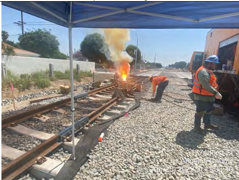
Wheeler to A St—FRT Thermite welding
