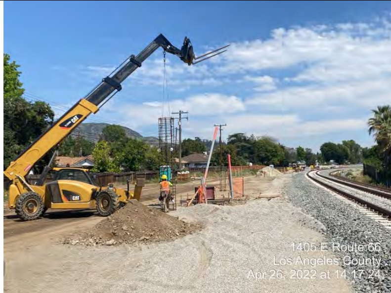
Loraine to Route 66— OCS foundation
