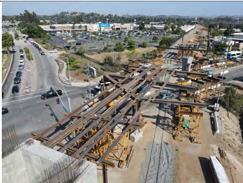
Lone Hill - Falsework
