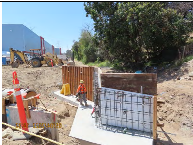
Route 66 to San Dimas wash-retaining wall work
