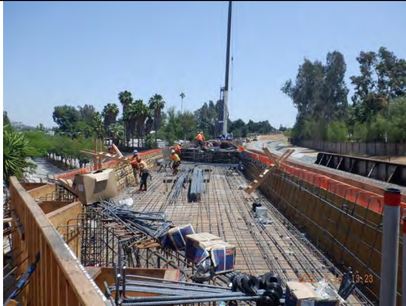
Route 66—LRT Structure
