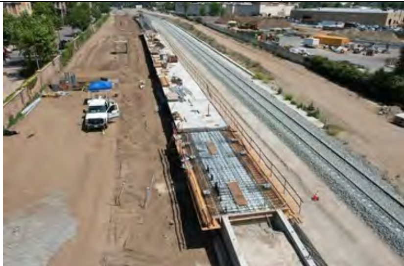
Glendora Station – Platform Deck
