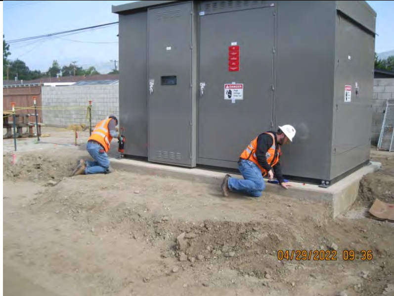
Loraine TPSS—Switch gear anchor bolts
