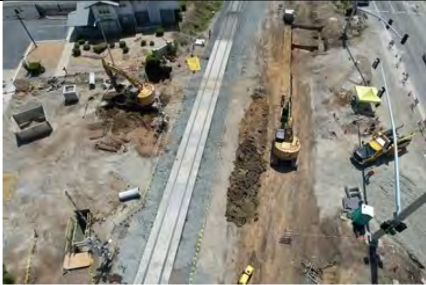
San Dimas Canyon Rd. crossing reconstruction
