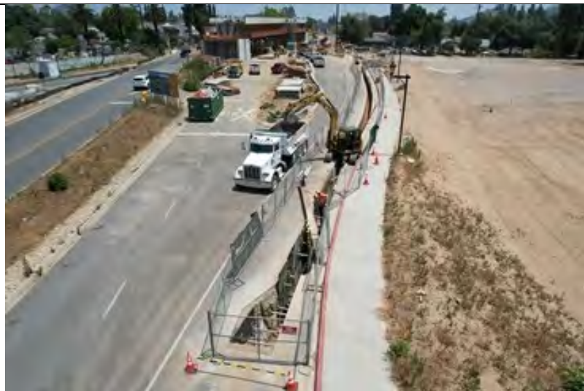
Bonita Cataract Ave. crossing - SoCal Edison power line relocation
