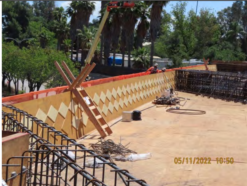
Route 66 — Stem wall formwork
