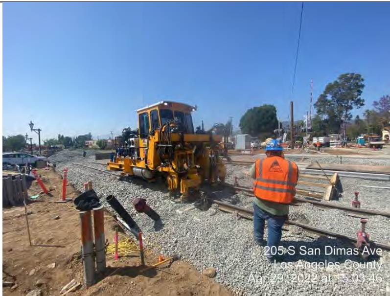
San Dimas Ave—LRT track tamping
