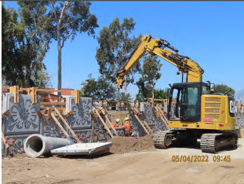
Foothill Grand to Vermont—MSE wall panel installation
