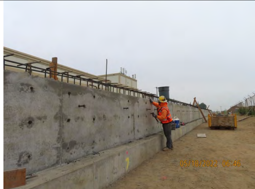
La Verne Station — Wall Finish work
