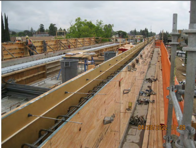
Bonita Cataract—LRT Structure
