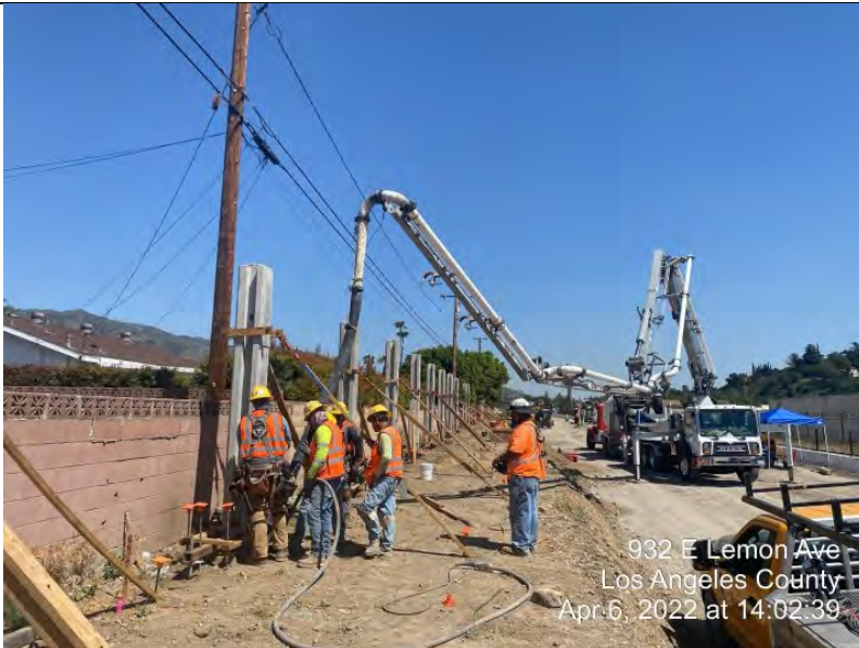
Elwood to Loraine— Soundwall Pilaster
