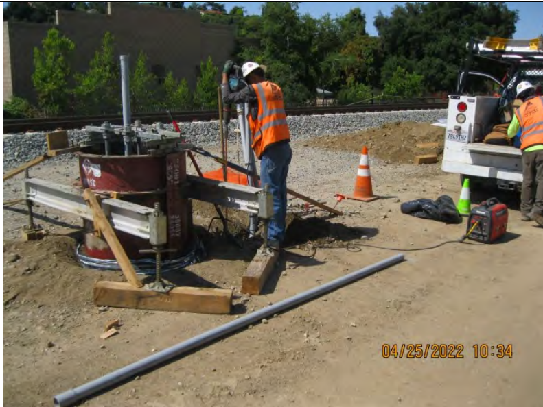
Loraine to Route 66— OCS foundation grouting
