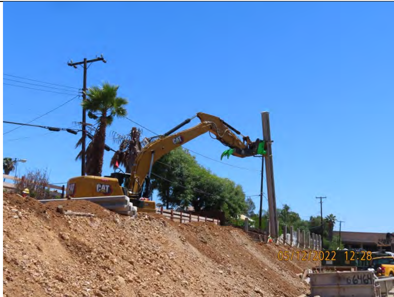
Route 66 to San Dimas Wash—Soundwall Pilaster
