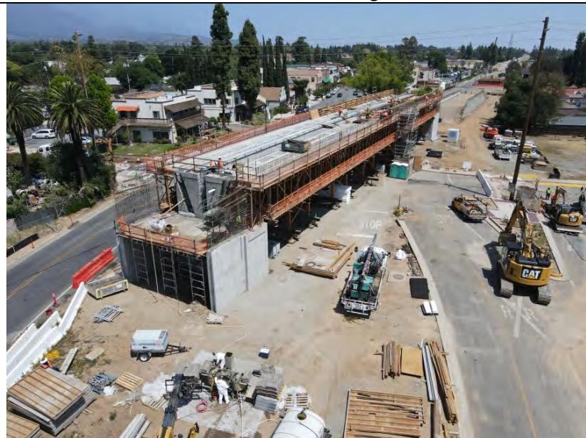
Bonita Cataract—LRT Structure
