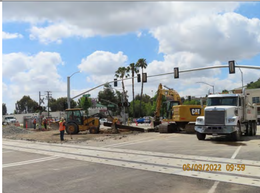
San Dimas Canyon — Demolition
