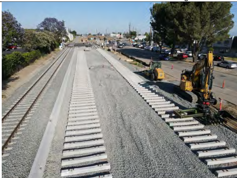
D St. to E St.—LRT Track Build
