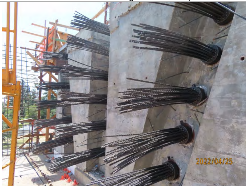
Bonita Cataract LRT - Tension cable
