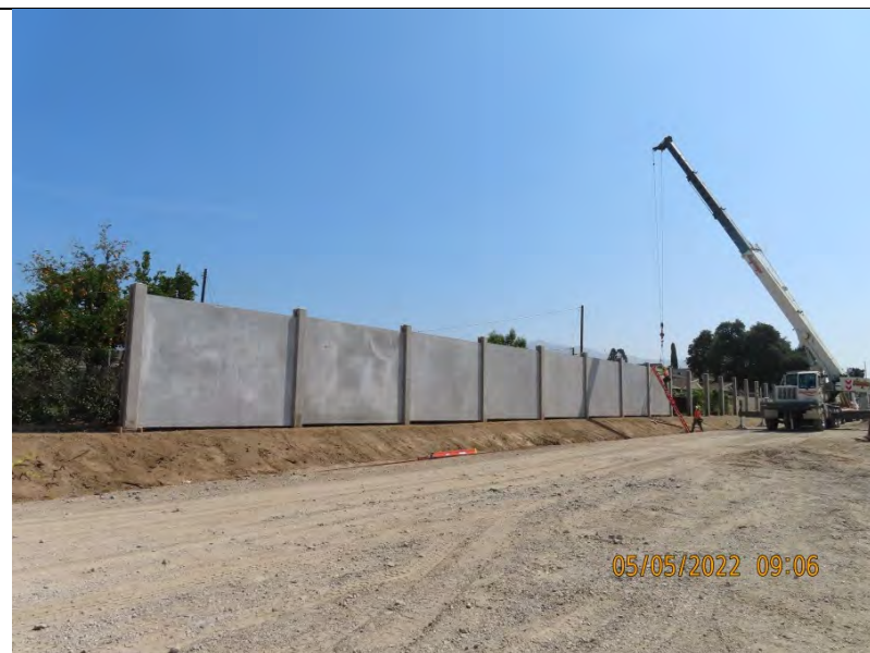
Pasadena to Glenwood—Soundwall
