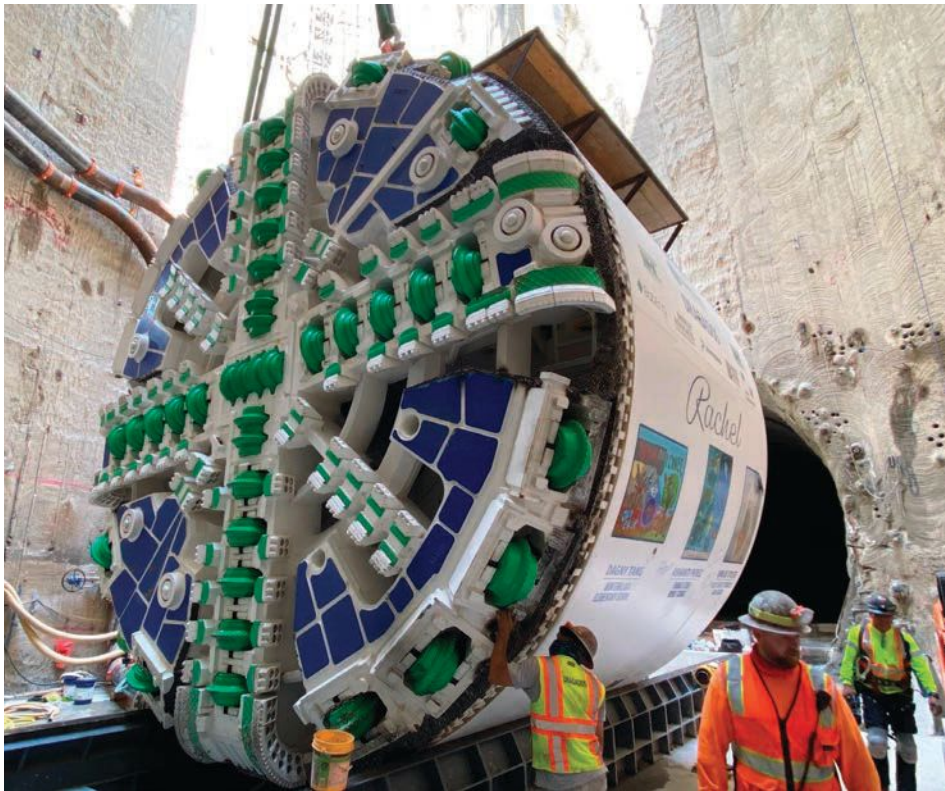
At left, tunnel miners move concrete tunnel wall segments to the tunnel boring machine (TBM) for placement in the Clearwater Tunnel. Below left, Sanitation Districts' General Manager Robert Ferrante and Sanitation Districts' Chairperson and Whittier Mayor Pro Tem Cathy Warner unveil the TBM decorated with student artwork. Above and at right, the TBM cutting head is lowered into the 135-foot-deep starting shaft to begin tunneling.
