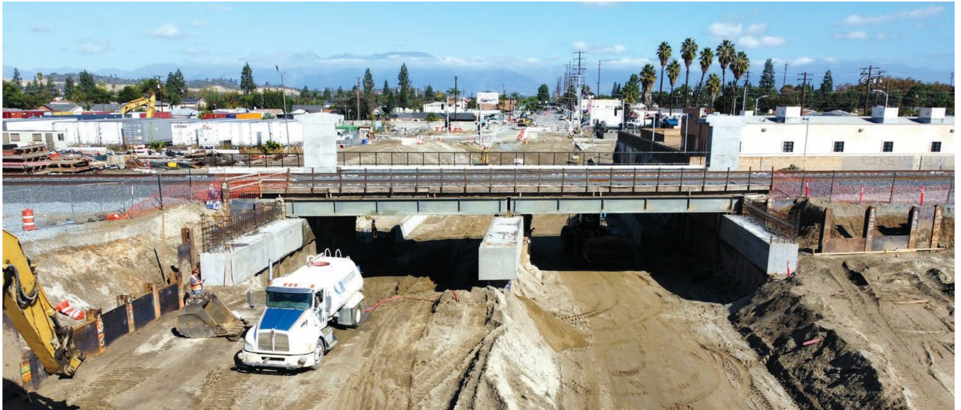
Far left, crews erected steel girders that will support the future four-track railroad bridge for the Fairway Drive grade separation in the City of Industry. Forty-nine trains pass through the railroad crossing daily. At left, the retaining walls under construction along Gale Avenue will support the roadway underpass for the Fullerton Road grade separation in the City of Industry. The project will enable freight trains to travel over Fullerton Road near State Route 60, preventing motorist delays and highway-rail conflicts. Above, the new railroad bridge and underpass are taking shape as crews continue excavation for the Durfee Avenue grade separation in Pico Rivera. The project will eliminate delays for emergency responders and the potential for vehicle-train crossing collisions.
