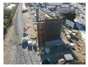
The Lone Hill Ave. bridge will be the largest bridge on the 9.1-mile project from Glendora to Pomona. When completed, the bridge will span 344 feet from abutment to abutment. The superstructure will have a minimum vertical clearance of 24 feet to allow freight trains to travel underneath. This is the one location between Glendora and Pomona where the freight system will switch from south to north positions in the corridor to continue serving customers.
