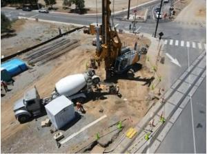
Other Bridge Work: Work has started on more than half of the 19 bridges to be built or renovated as part of the project. At the intersection of Foothill Blvd./Grand Ave. in Glendora, crews continue to make progress building the retaining walls of the western approach for the future light rail bridge that will carry Gold Line trains over the intersection. As seen in the photo below (left), the walls for the approach will consist of custom form panels that feature the project's citrus design.
