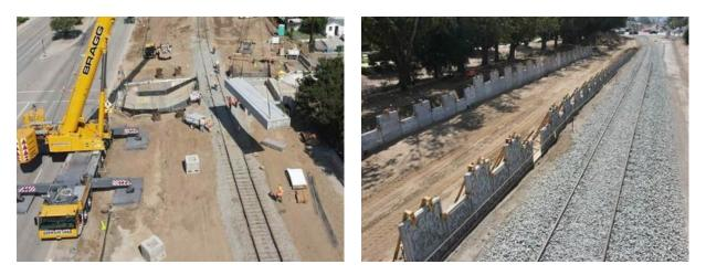
**Glendora Station Update:** At the site of the future Glendora station, crews have now completed the major structures for the pedestrian undercrossing that will provide riders access to the station platform. As seen in the photo below, the walls of the ramp to the station platform have been completed. Future riders will walk up this ramp - seeing the citrus design patterns on the walls - and onto the Glendora Station platform to board the trains.
