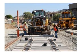
Photo (left): Crews install one of the two new light rail tracks at the Glendora Ave. grade crossing. The crossing has undergone extensive underground utility work, requiring the street to be closed since August.
