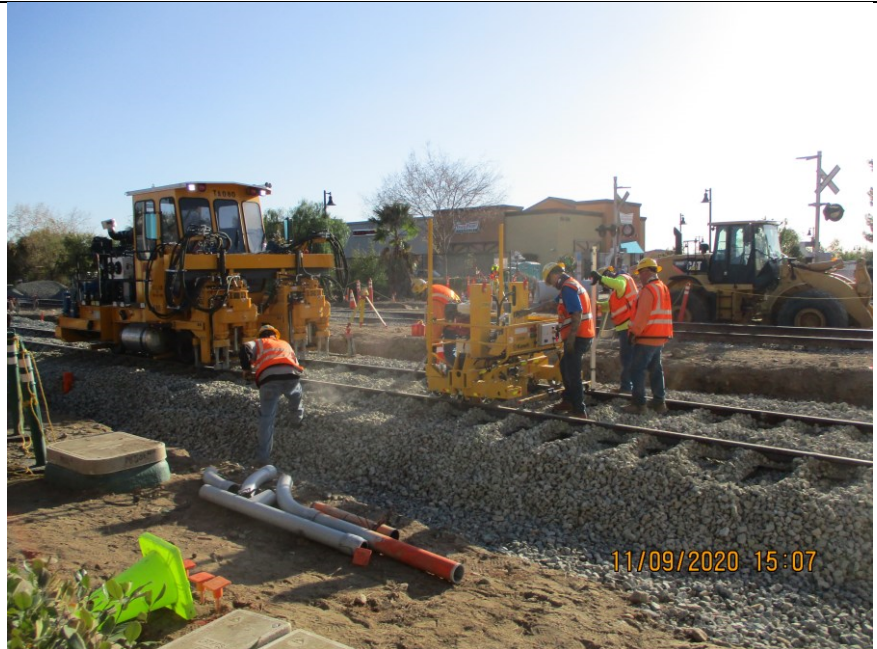
Gladstone—FRT track alignment and tie tamper
