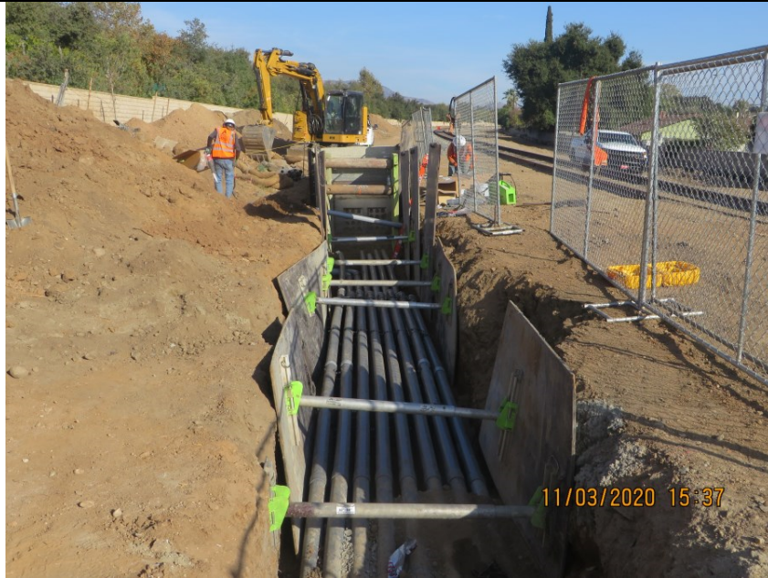
Barranca—Ductbank placement
