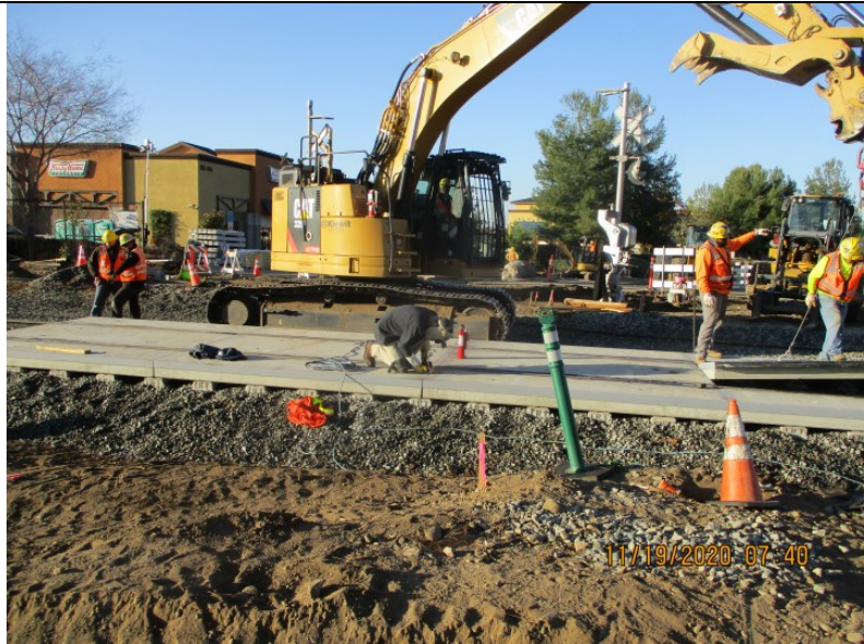
Gladstone - LRT Track panels welds
