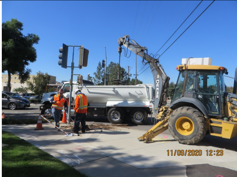
Wheeler - Traffic signal pole foundation auger
