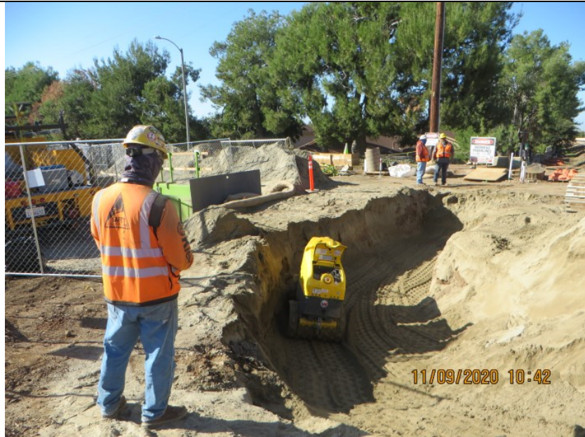
Barranca—Storm drain backfill compaction
