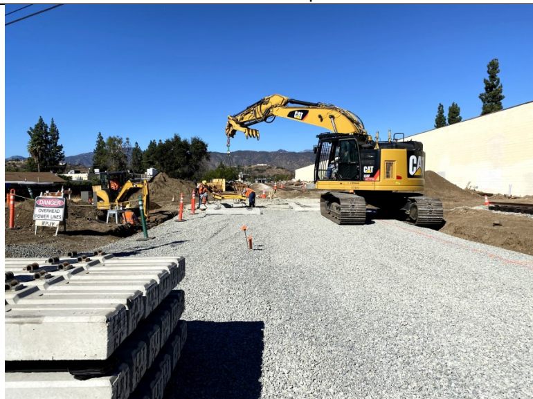
Gladstone - LRT track tie placement
