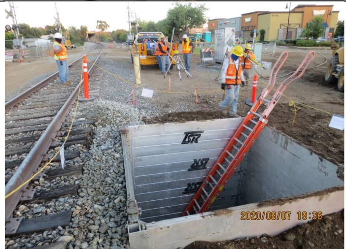
Segment 2A: Gladstone Trench box for LRT ductbank pullbox installation
