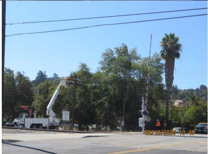
Segment 1B: Freight abandoned pole line removal
