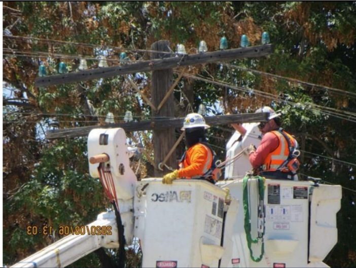
Segment 1A: Freight abandoned pole line removal
