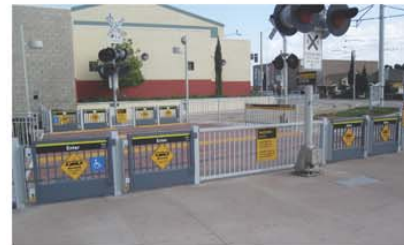
Pedestrian Grade Crossing Gates and Flashers
