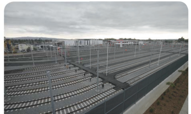
Most of the nearly six miles of track installed at the Campus will be used for storage of up to 84 light rail vehicles when not in use.
