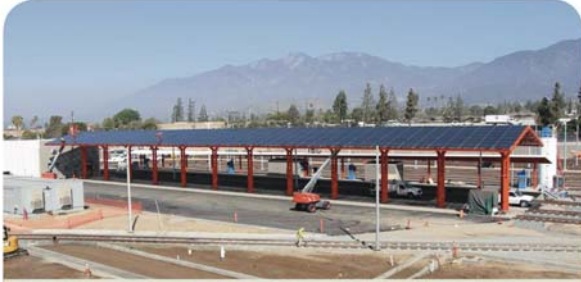
A solar panel array atop the Maintenance of Way canopy will provide nearly 33% of power needed for the 132,000 square foot Main Shop Building.
